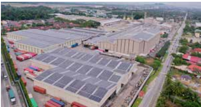
Aerial view of Solar PV System in Penang
