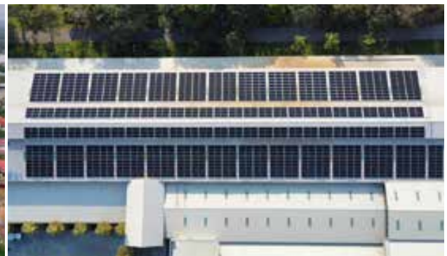
Aerial view of Solar PV system in Melaka
