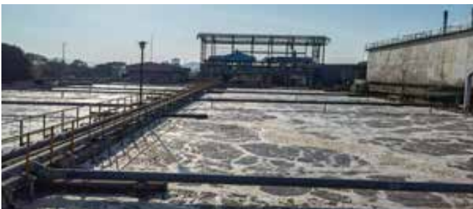
Water treatment plant in Kajang
